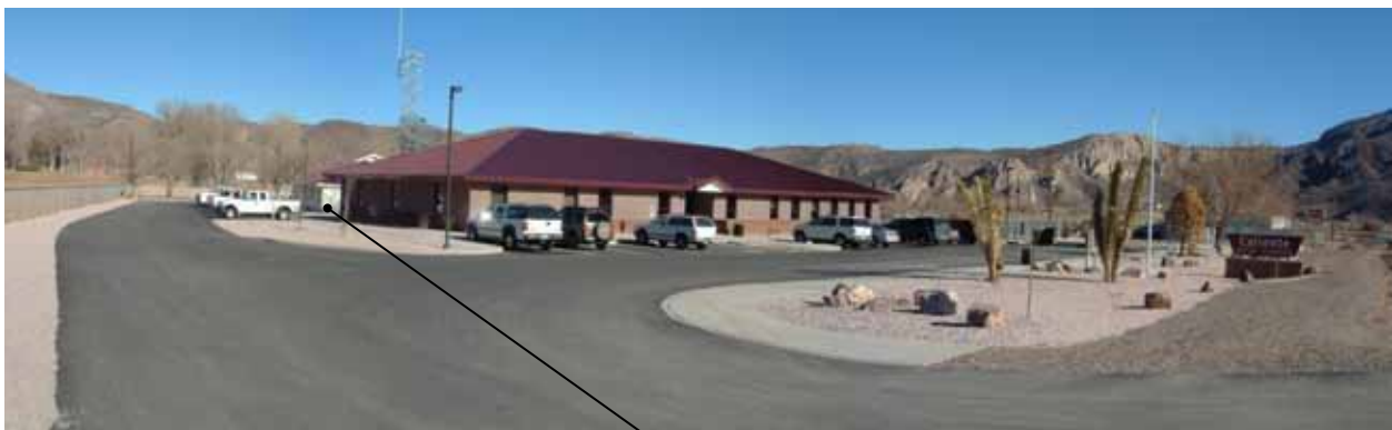
Caliente Maintenance Wareyard, Nevada
