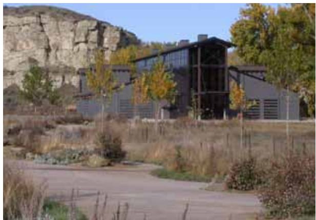
Pompeys Pillar National Monument Interpretive Center, Montana
