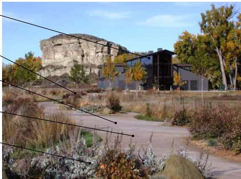
Pompeys Pillar National Monument Interpretive Center, Montana
