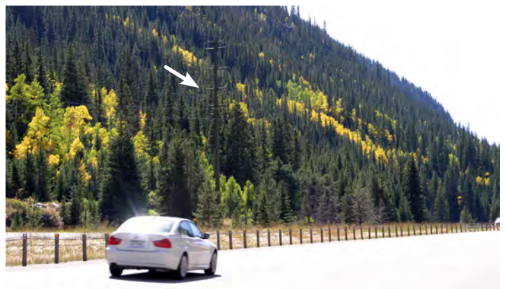
Transmission power line that was factory painted with a single color and installed circa 1976.
