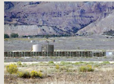
A stand-alone fiberglass screen blocks the view of a well pad. The pattern can be customized to better match the landscape. Photo credit: www.LBIE.com
