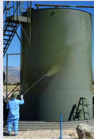
Apply the base coat.
