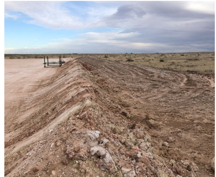
Topsoil stockpile located on east side of well site; Three-foot berm on east edge of well site
