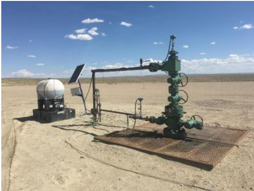
Wellhead with adequate cover over cellar; Chemical tank with adequate catchment
