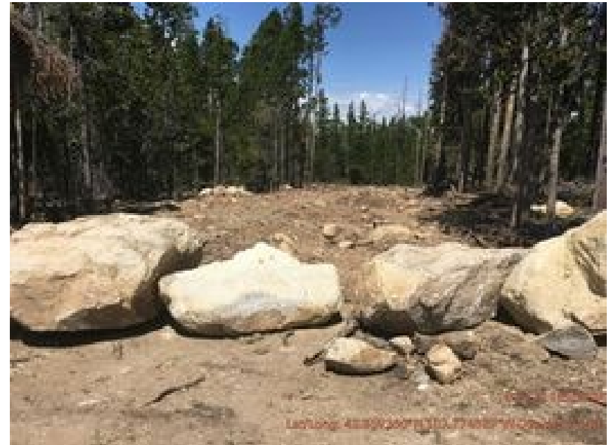
Boulders blocking reclaimed access road; COA requirement
