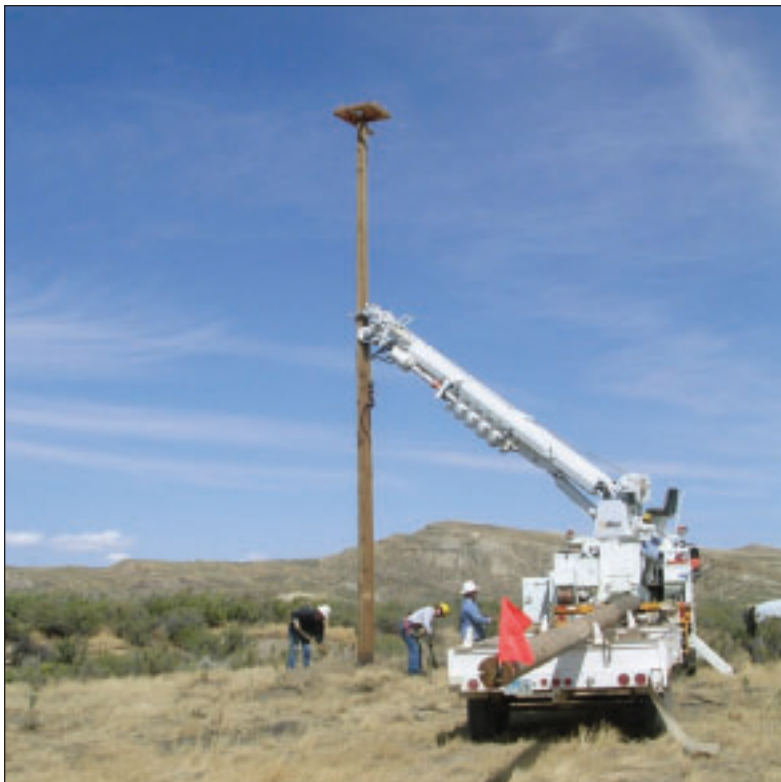
FIGURE 7.1: Utility crew installing raptor nest platform.
