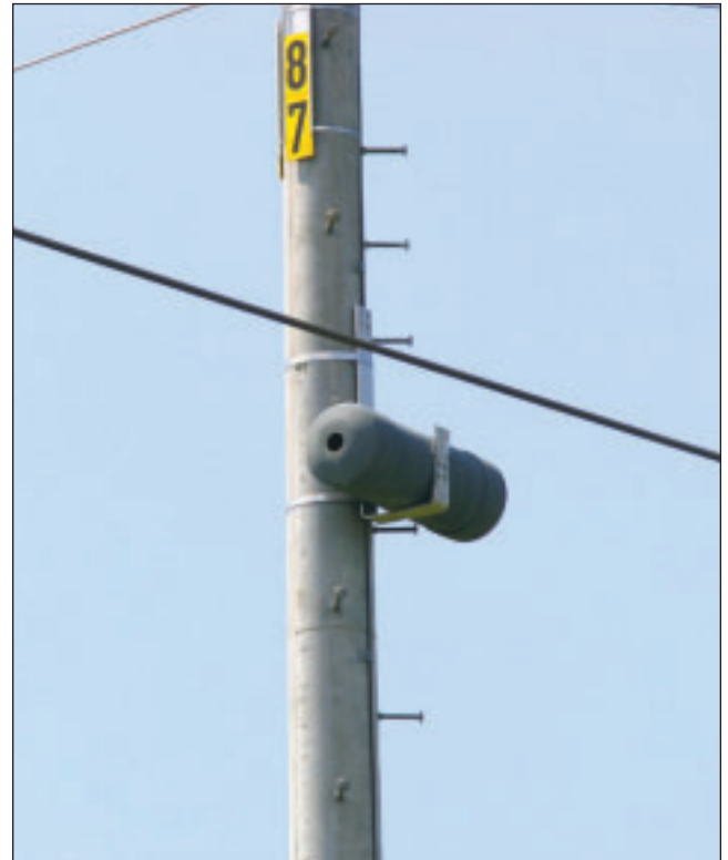
FIGURE 6.19: Kestrel nesting tube (91-cm [36-in] length) installed on transmission tower in Georgia.
